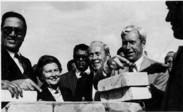
Egypt's Nagy Shalla, Mrs. Betty Atherton, Ambassador Alfred L. Atherton, Jr. and AID's Michael Stone at start of construction of new school in the village of Fedan El-Feki. (Photo by Khaled Abou Seif)
